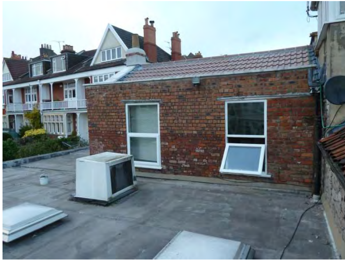
Plate 8. The flat roof of the single storey and rear 1 st floor.
