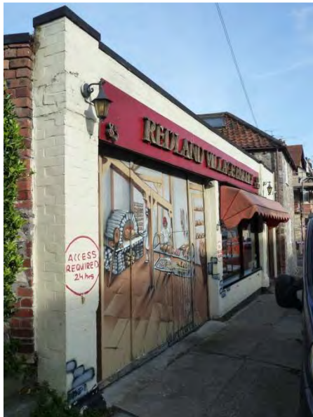
Plate 2. The brick frontage and double door vehicle entrance.
