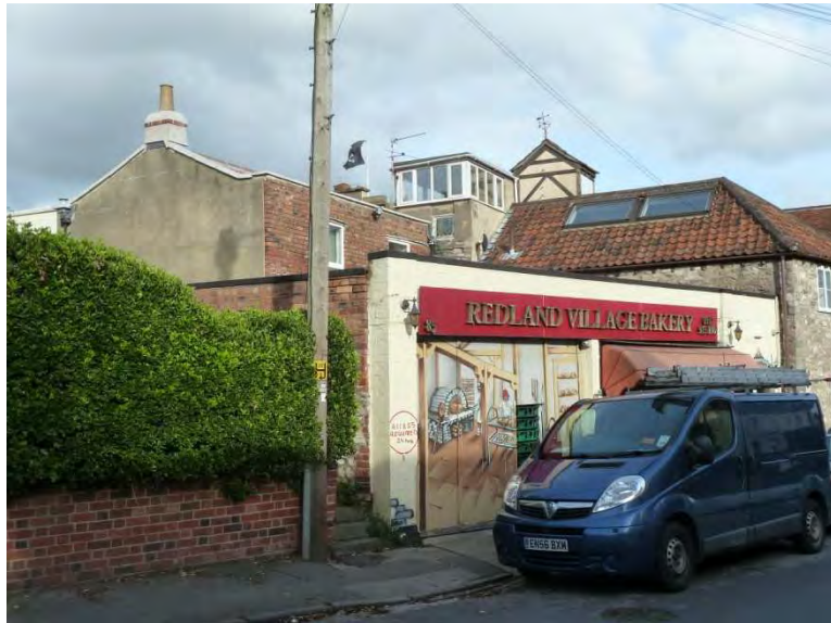
Plate 1. The frontage, rear two storey and adjacent 'Ye Olde Cottage'.
